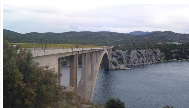
The bridge seemed much longer than it looks here
