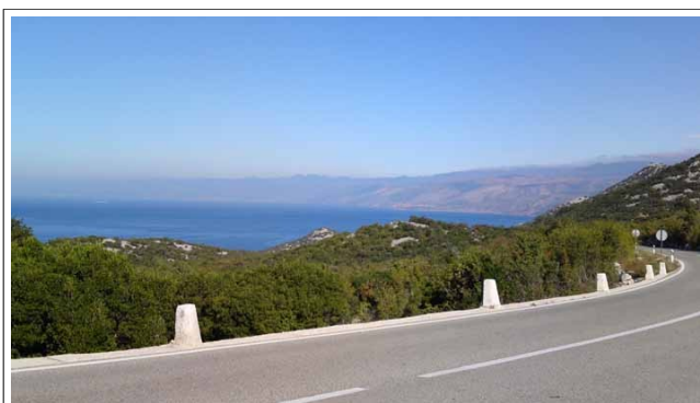
Great views, sheer drops and no barrier!
